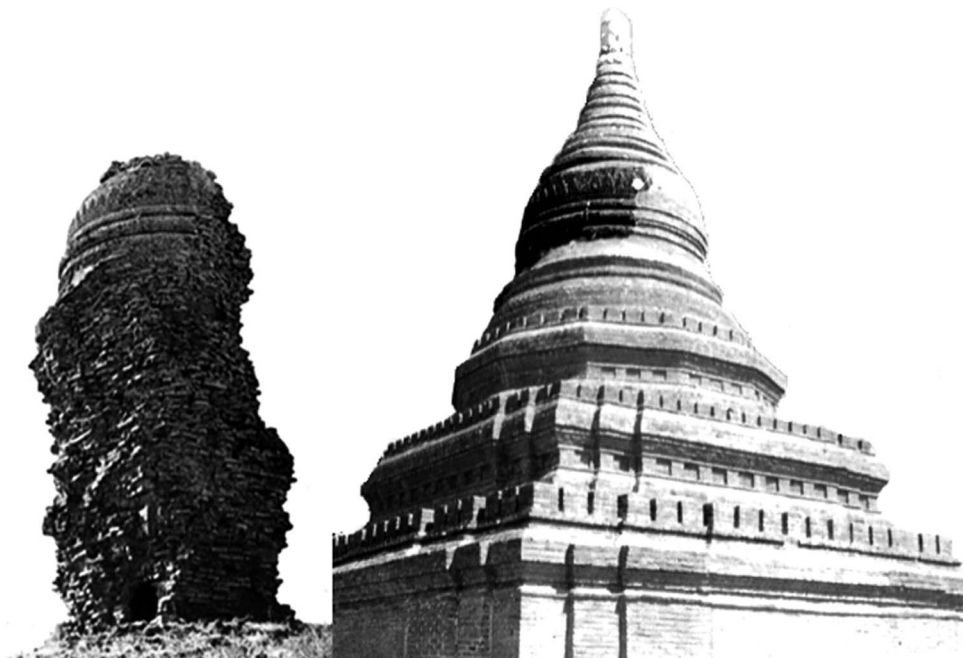
Plate 1 Stupa 770 before (left) and after (right) reconstruction in 1997.
